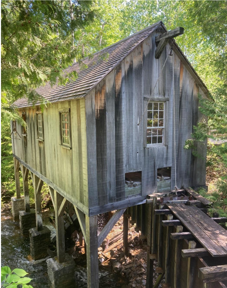
Outside of sawmill. The sluice feeds the head water under the mill. Opening the sluice gate (attached to the rope) allows the water to flow down to the wheel.
