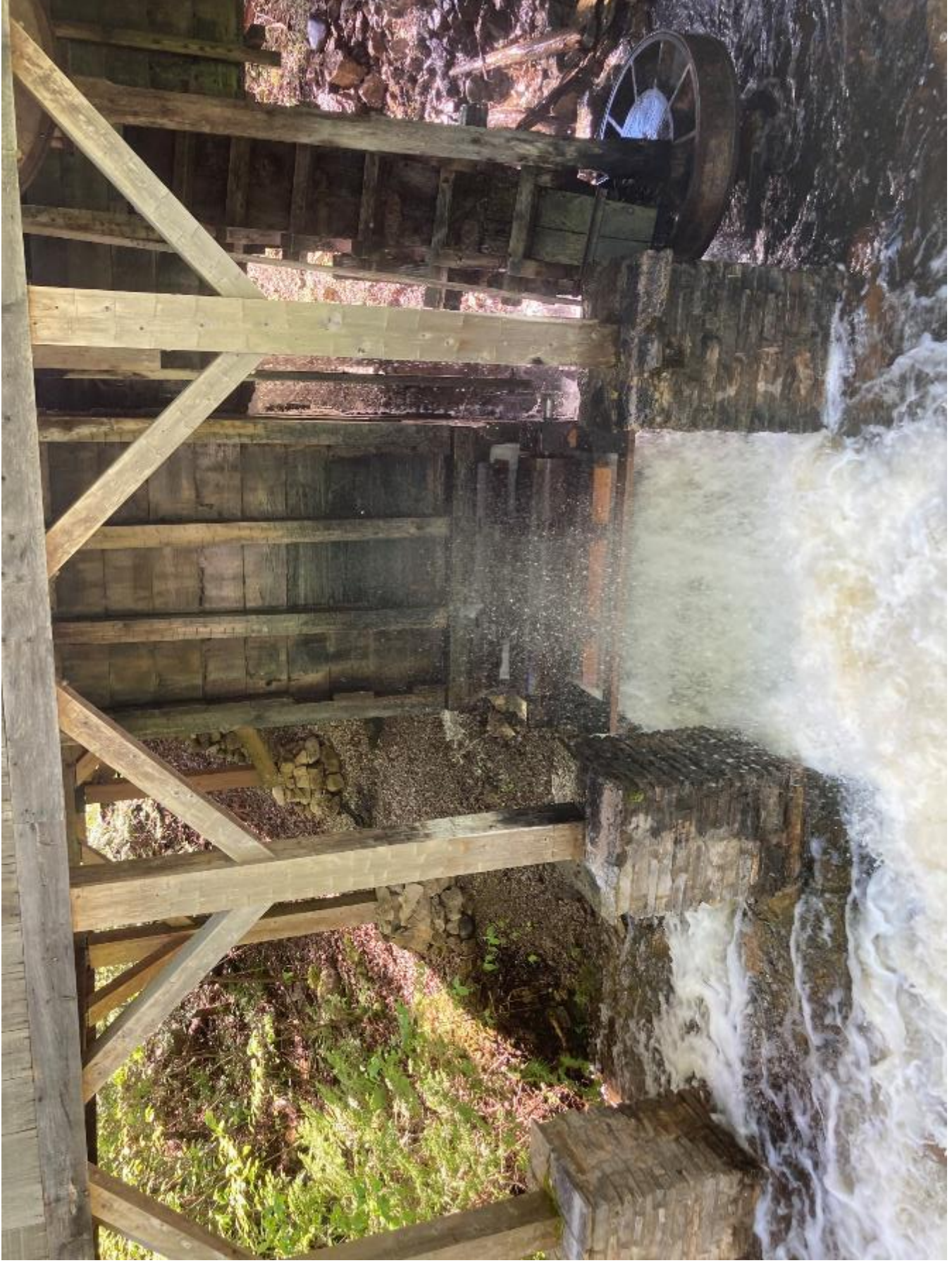
Tail water exiting the sluice chute while turning the flutter wheel.
