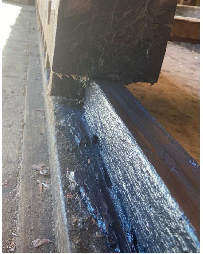
Wooden beams used as ways for the carriage. Heavily greased.
